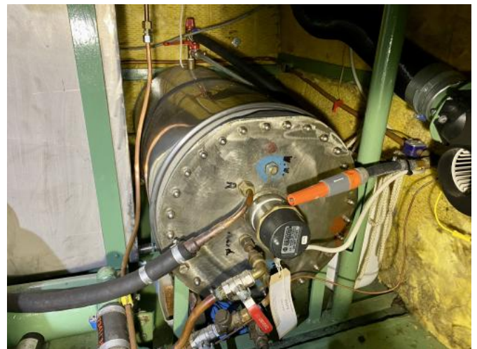
Warmwasserboiler
